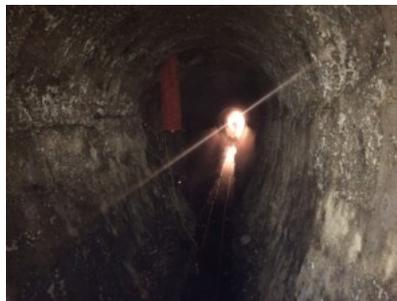
*Sade Canada based out of Quebec City mobilized to Winnipeg to access both Trunk Sewers and complete pre-manufacturing surveys. This was completed manually, by taking measurements every 1m of the height and width of the sewer.*
