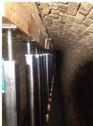
*The crown of the sewer, approximately 15m (50ft) from the downstream manhole, had settled/dropped approximately 70mm (3 in) requiring temporary bracing to be installed.*
