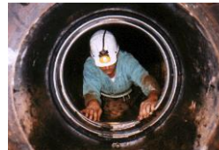
Install Retaining Bands
