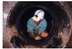
Install Rubber Seal
