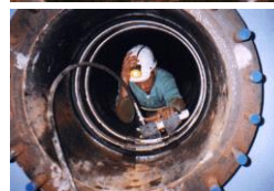
Expand Bands with Expander
